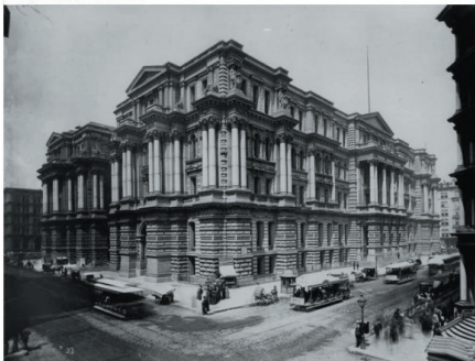
Chicago City Hall and County Building, built 1885. It suffered from structural defects with its foundation that caused the building to sink, and was later replaced with the current City Hall in 1911.
