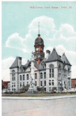
Will County Courthouse, Joliet, Illinois (Built between 1884-1887); Demolished
